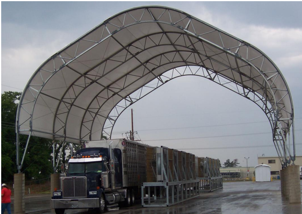
Figure 5b. Canopy and bank of cooling fans in waiting area at the plant
