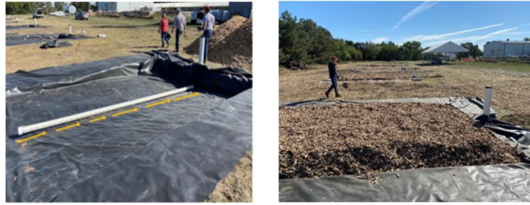
Figure 2. Leachate collection system and wood chip base in disposal units
