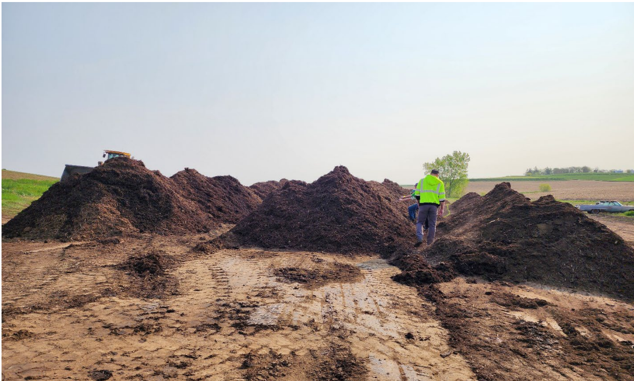
Photo 4. Windrows nearing completion of construction (Flory).
