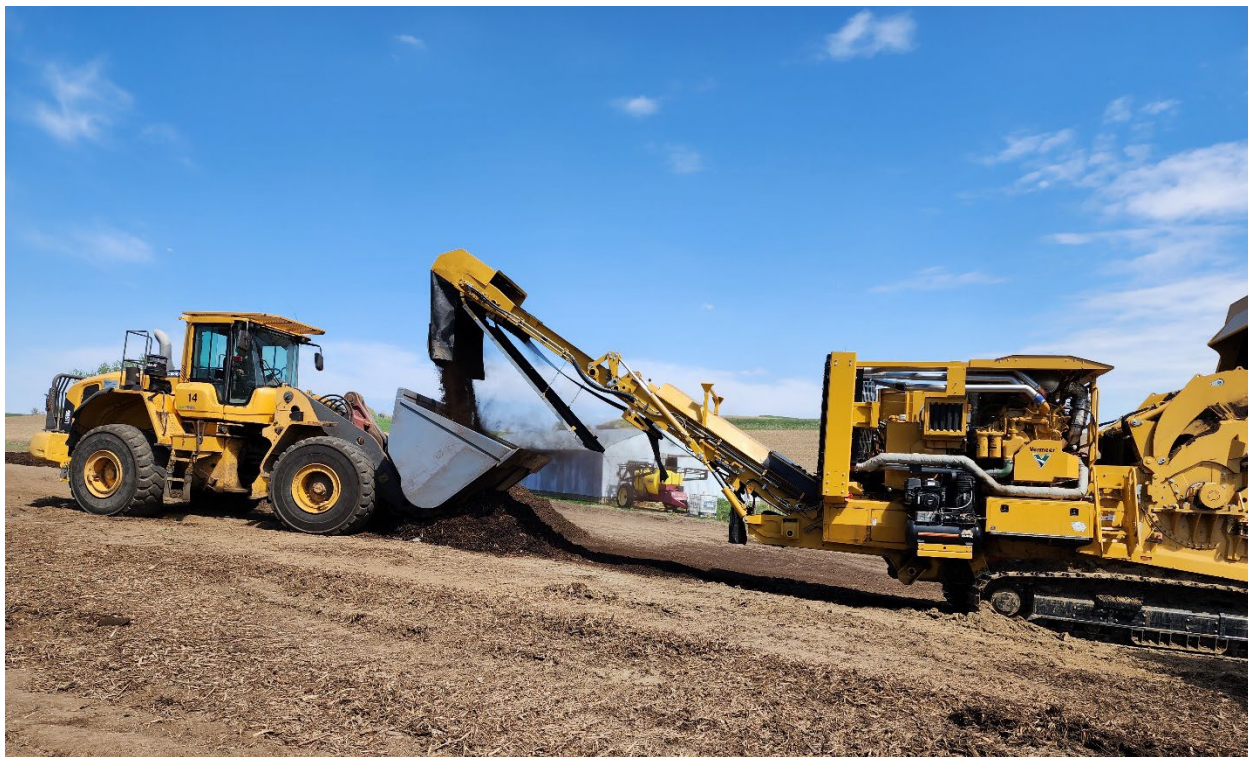
Photo 2. Excavator, grinder, loader (Flory).
